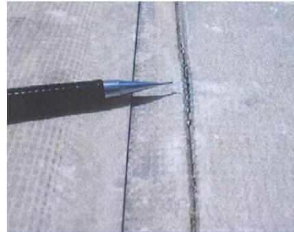
Figure 6: Aged TPO Membrane Problems
